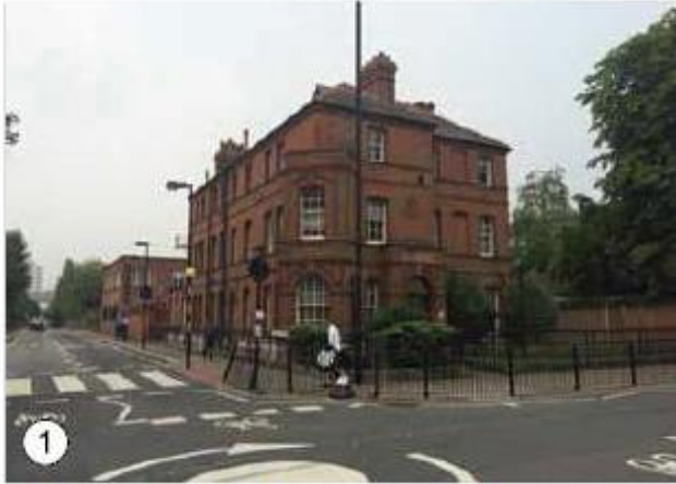
1 View of St. Ann's Police Station from St. Ann's Road, looking down Hermitage Road
